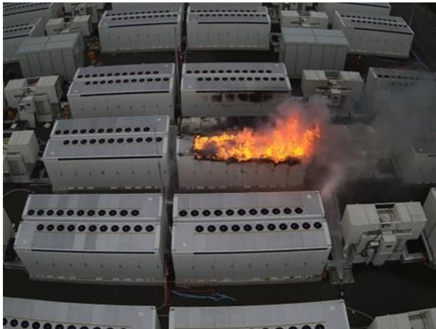
Figure 34 Two of Australia's shipping-container-sized battery packs going up in smoke https://www.ans.org/news/article-3292/australia-has-invested-in-batteries-for-grid-security-its-not-going-as-planned/
