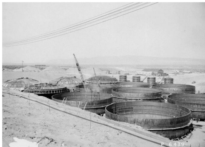
Figure 80 Hanford's waste tanks during construction (typically 1 million gallons each)
